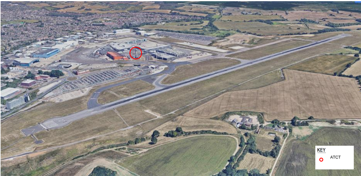
Figure 4-2 Existing Site Context Aerial Photograph (Source: www.google.com/maps)
